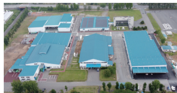
Our production facility under expansion (Kitakami, Japan)
