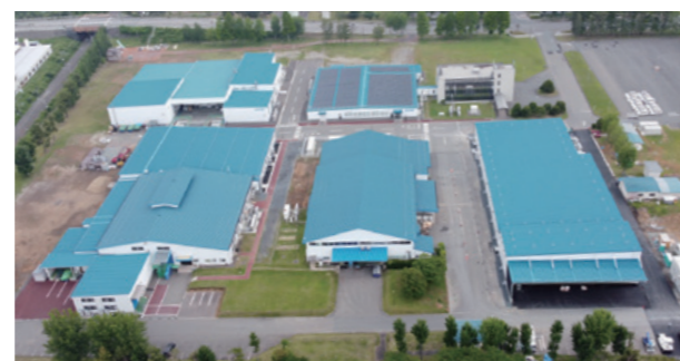
Our production facility under expansion (Kitakami, Japan)
